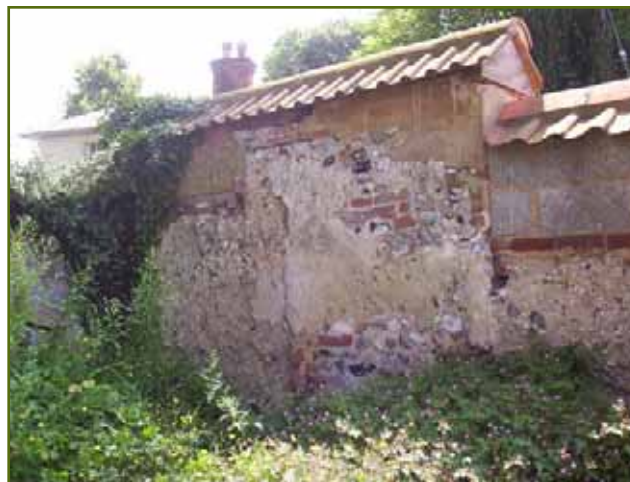
Figure 5 Cob walls with 'Bridgewater' interlocking tiles
